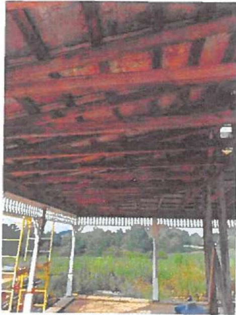
Photo taken 8/10/22 of front porch roof being installed
