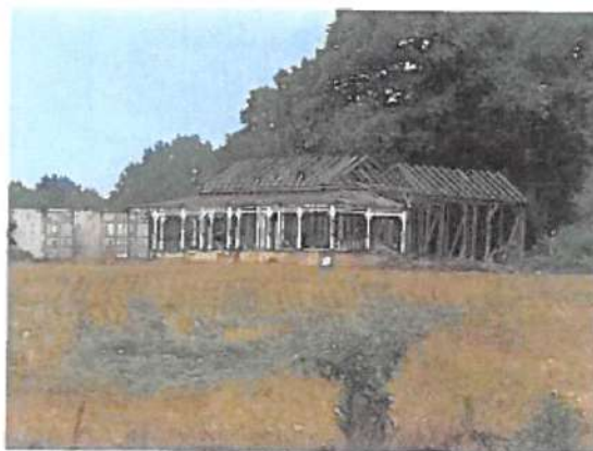
Photo taken 7/8/22 of overall house structure
